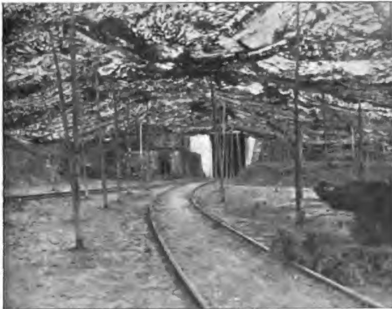
CAMOUFLAGED ENTRANCE TO EMPLACEMENT FOR 340-MM. FRENCH GUN (CONSTRUCTED BY AMERICANS).
